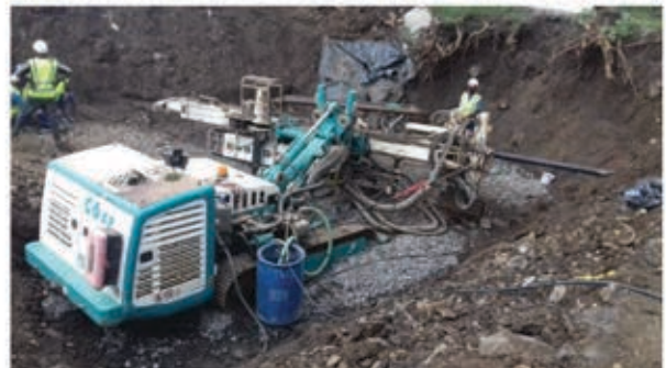
Casagrande C6XP installing horizontal anchors
